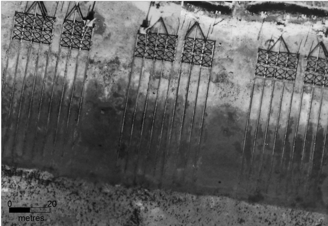
Figure 11: Extract of RAF aerial photograph RAF/106G/UK/955/RVp3/6246 30-OCT-1945 showing detail of the slipways with the raised trellis or platform with the possible winch housing and tether points at the top of the beach. Historic England Archive RAF photography.
