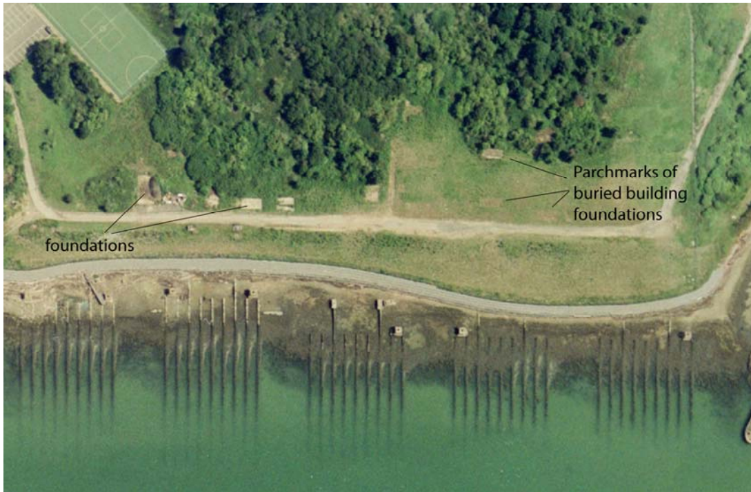
Figure 15: Extract of Google Earth aerial photograph dated 01-JAN-1999 (though vegetation suggests a summer date) showing surviving steel and concrete remains of the D-Day slipways. It also shows the remains of the concrete hut bases and parchmarks of further buried foundations, hard-standings and roads of the Second World War maintenance yard located above the beach on Horsea Island. EARTH.GOOGLE.COM ACCESSED 04-FEB-2020.
