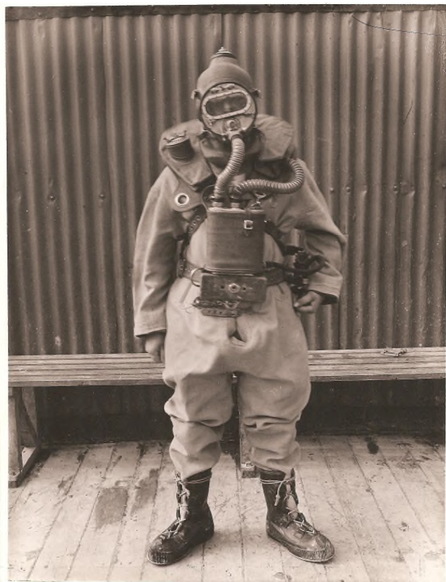
'Port' Party diving suit with self contained breathing apparatus, specially developed for D-Day operations. All non-magnetic.
