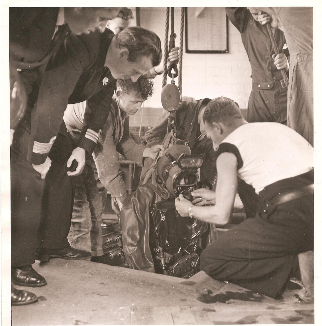
Unconscious diver, under supervision of the medical officer, being removed from the 'wet pot' during tests on breathing mixtures before D-Day Normandy Landing.
