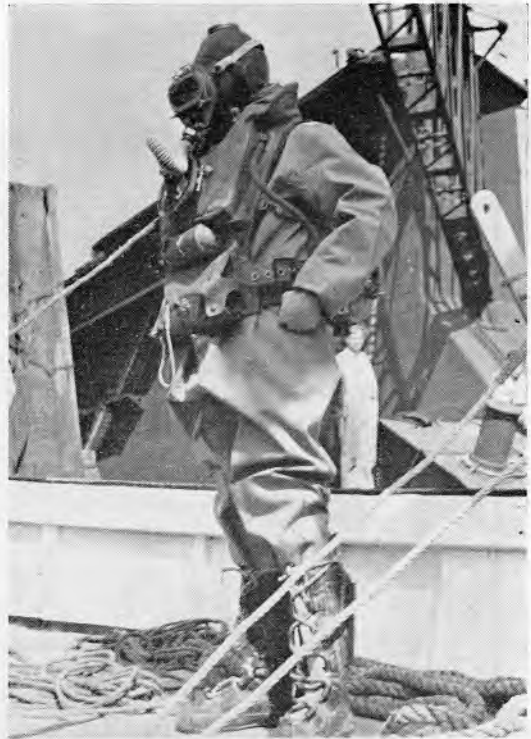
Chatham 1953. Diver dressed in A.S.W.D.D. and C.D.B.A. 5561A. Diver has hand on his bypass valve
