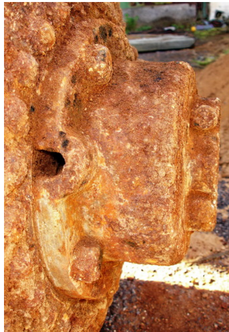
The external gland arrangement on the base of the mine.
